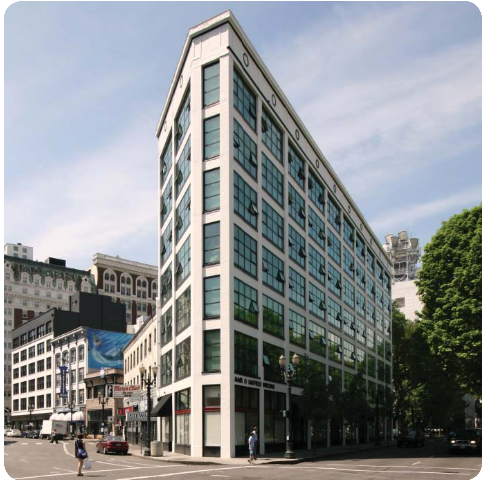
Hatfield Building in 2012, window replacement and exterior work complete, corner of West Burnside & Broadway Streets source: Central City Concern
