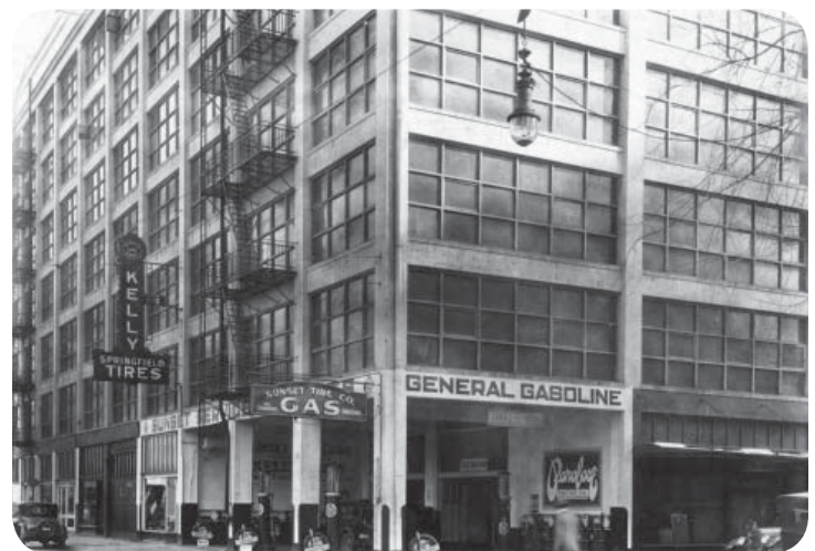
Hatfield Building in 1928, then known as the Lowengart Building, corner of 8th Avenue & West Burnside Street before north 20' portion of building was removed in 1931 to widen Burnside Street. source: City of Portland Archives, Oregon, A2000-033.
